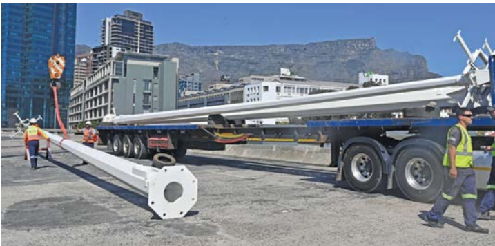
In pole position: Central Cape Town is about to be seen in an even brighter light as 85 high-mast streetlights are up for refurbishment and LED retrofits.
