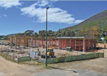
Wastewater works in for a treat: The Wildevloëlvlei wastewater treatment plant, which serves Fish Hoek, Kommetjie, Noordhoek, Ocean View and Masiphumelele, is undergoing a multimillion-rand upgrade.
